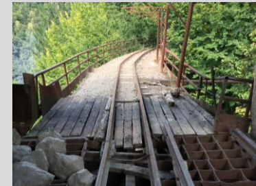
1km tramway to processing plant
