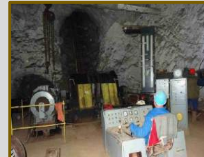
Underground hoist chamber
